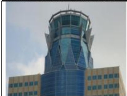
Physicians Office Tower Crown Custom Curtain Wall
