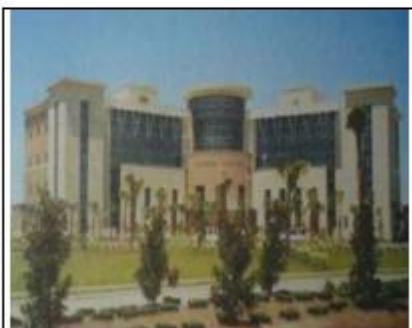
Galveston County Justice Center Hurricane Impact Curtain Wall
