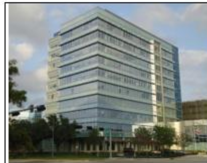
Toyota Business Center Unitized Curtain Wall
