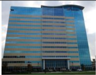
CEMEX Office Tower I Beam Curtain Wall & Strip Windows
