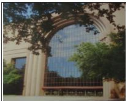
Worham Worham Theater Overhead Suspended Curtain Wall
